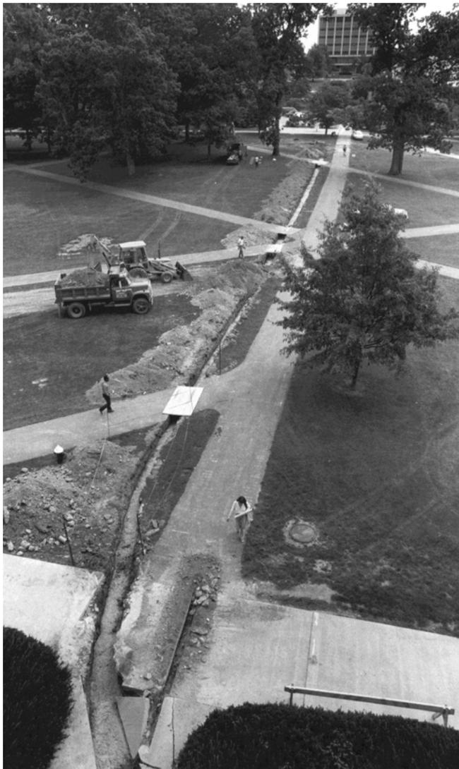
Figure 9. Telecommunications cable being laid on the Arts Quad
