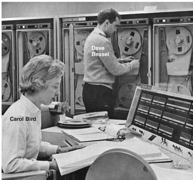
Figure 1. Control Data 1604 console and magnetic tape units
